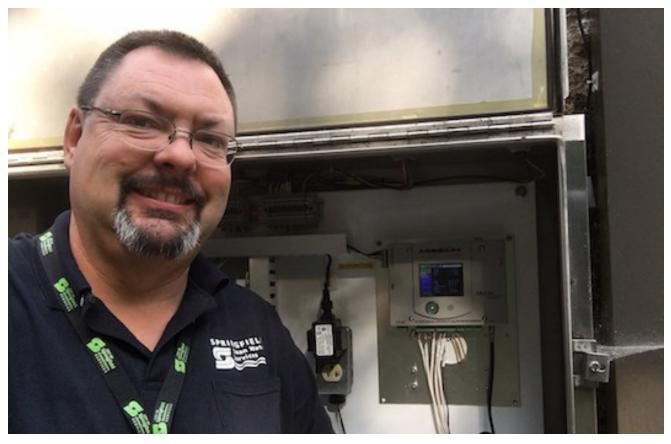
John Copelin said lightning struck the second largest pump station in Springfield on a Saturday, traveling up the solitary phone line for the alarm system, destroying the connection and terminating pumping at the station until the following Monday. Had the unit used a cellular connection, he said the line would not have been disconnected, and an alert about the station would have been sent.
