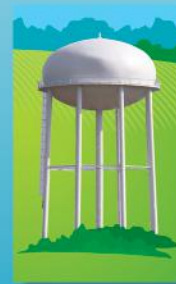
Tank and Well Control
