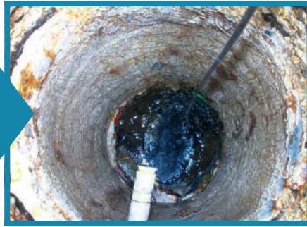
Left: Damaged manhole before rehabilitation work; Right: Manhole after repair
