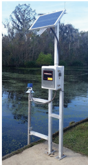
Solar application using 20 W solar panel
