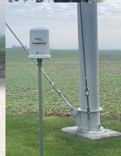
The Mission Tank and Well System maintains the water level in a storage tank by automatically commanding remote well or booster pumps to turn on and off. The system relies on standard Mission remote terminal units (RTUs) and a transducer to monitor the tank level. There are no private radio networks, computers or programmable logic controllers (PLCs) to maintain. It is low cost and easy to set up.
