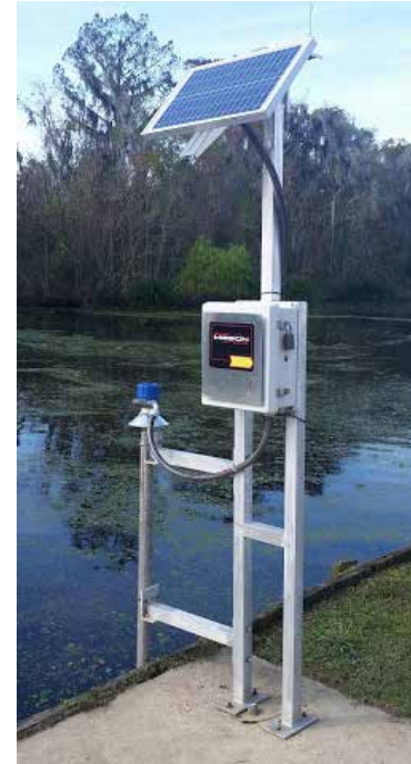
Solar application using 20 W solar panel
