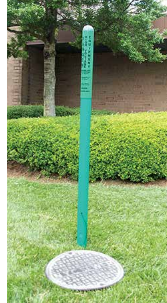
Manhole Monitor above-ground antenna
